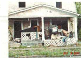
Excessive Rubbish/Trash Open/Vacant
